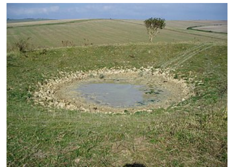
Dew pond at Cockroost Hill, parish of Portslade , Sussex , showing layer of chalk rubble protecting the lining
