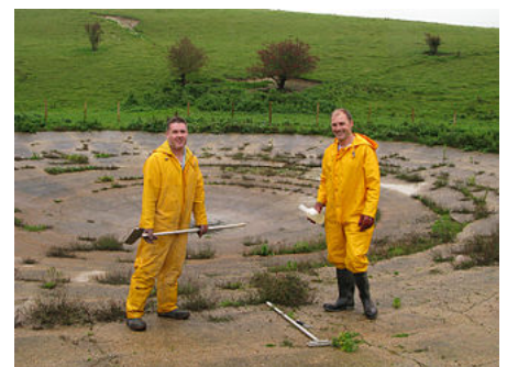
Modern examples made with portland cement need regular repair. [4] Oxteddle Bottom, Sussex
